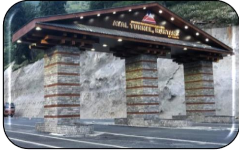
Atal Tunnel (Longest Highway Tunnel in the world- 9.2 km)
